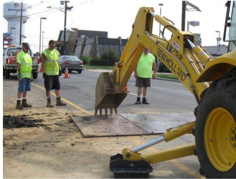
The excavation was covered with a road plate which was held in place by large spikes. Efforts to remove the spikes with hand tools were unsuccessful. The decision was made to use the backhoe to lift the plate allowing the spikes to be removed. The operator waited until workers were clear of the area before using the bucket to lift the plate. Again the individual ensuring that traffic did not intrude was not equipped with a traffic control device.
