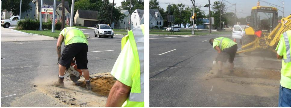
A cutoff saw was used to square the opening in the asphalt. This operation was completed without the use of water or any wetting method. Dry cutting of certain materials exposes workers to silica. This saw was equipped to be used with a water supply. According to workers, the water supply was not available for this job. The level of dust generated exceeded recommended PELs. (Permissible Exposure Limits)
